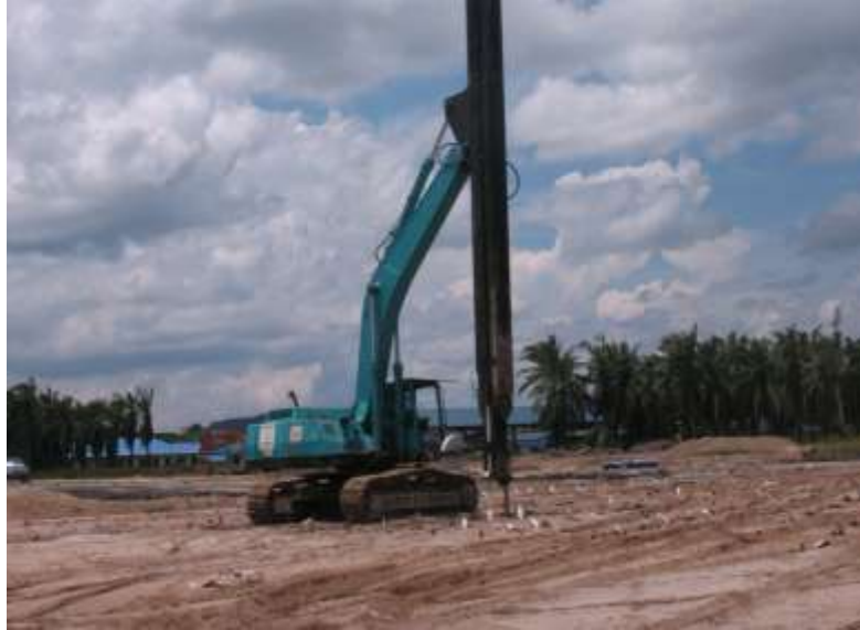
Figure 3: Installation of PVD prior to surcharge
