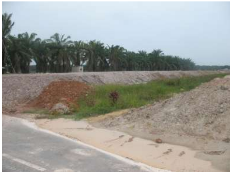
Figure 4: Complete Surcharge at Resting Period.
