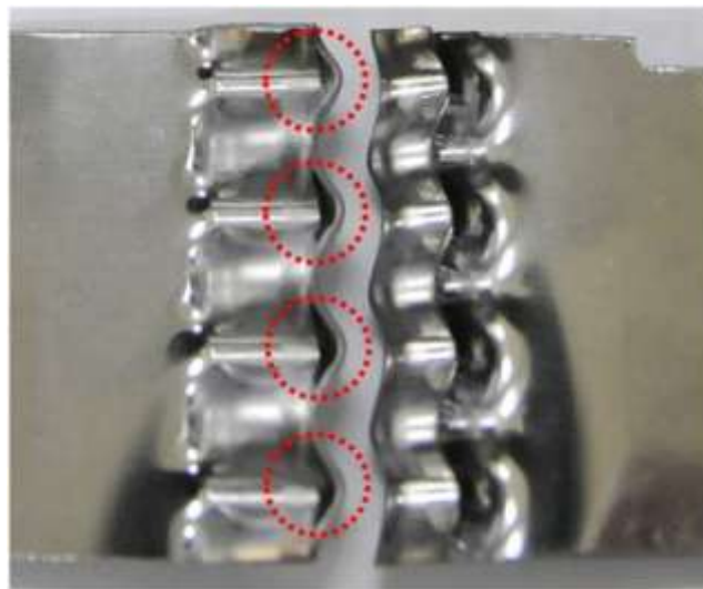
Fig. 4 The origin of crack in caulking part
